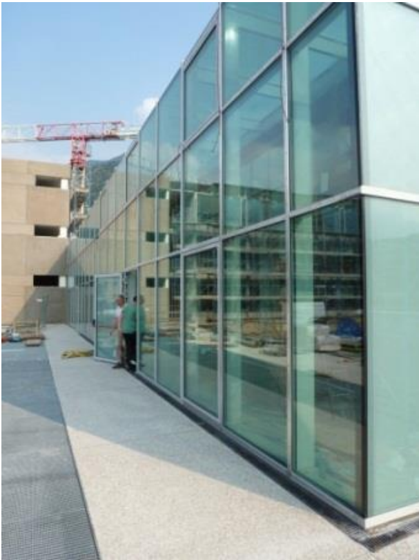
School of Romarzollo under construction
